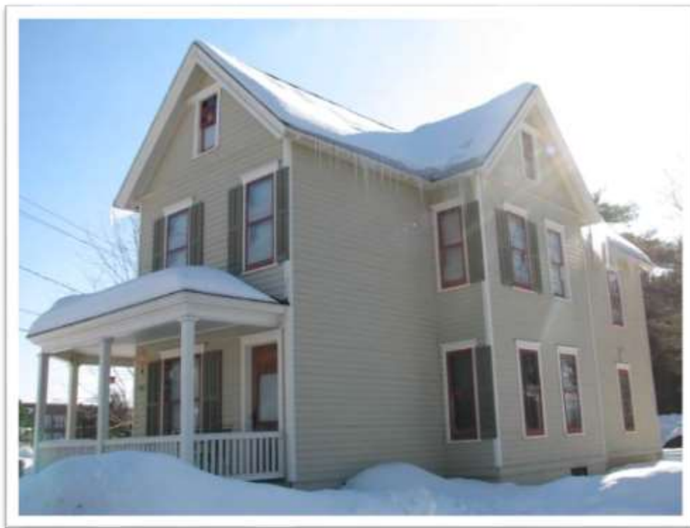
North Elevation (façade)
