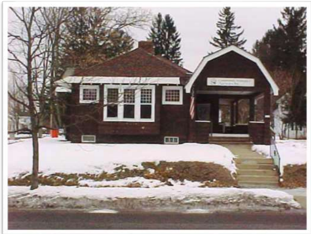
South Elevation (façade)
