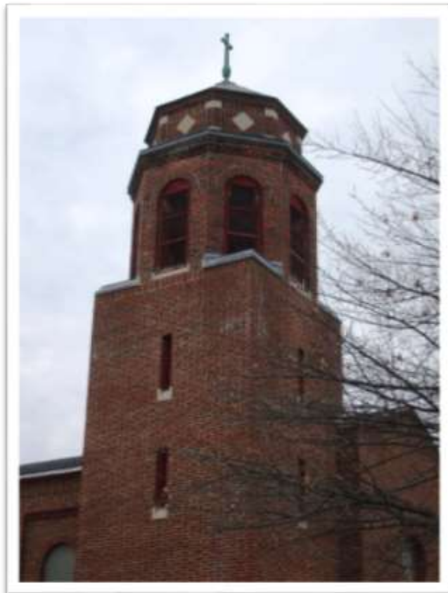
Bell tower on the northeast side of the church
