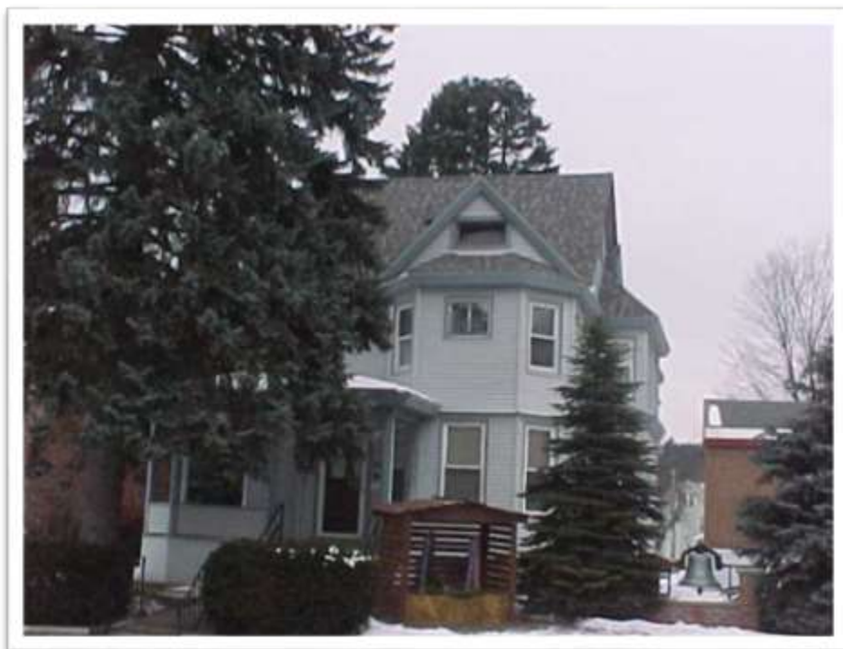
Olmstead House & Parsonage
