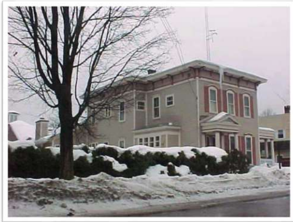
South Elevation (Façade)
