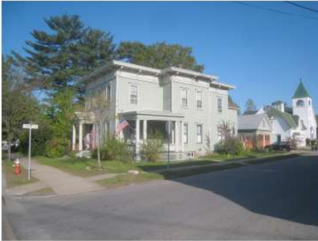
Southeast corner looking Northwest
