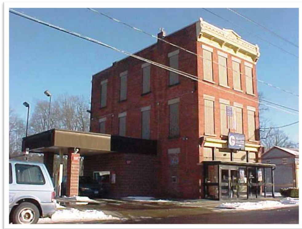
West (façade) and North elevations
