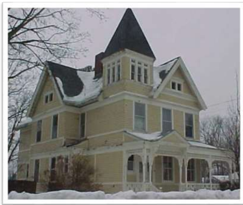
2006 Previous to renovations.
