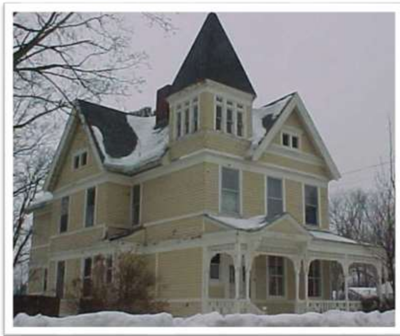
2006 Previous to renovations.
