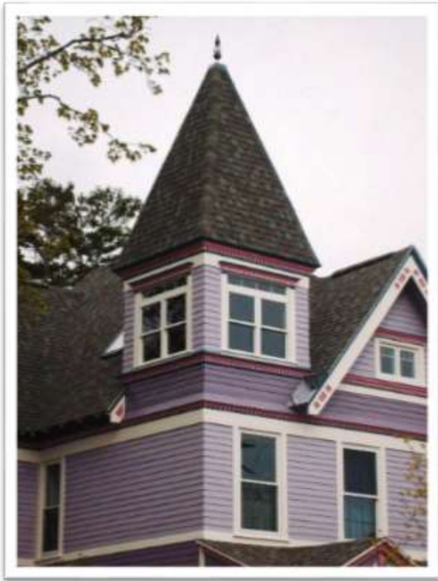
Note tower windows were replaced.
