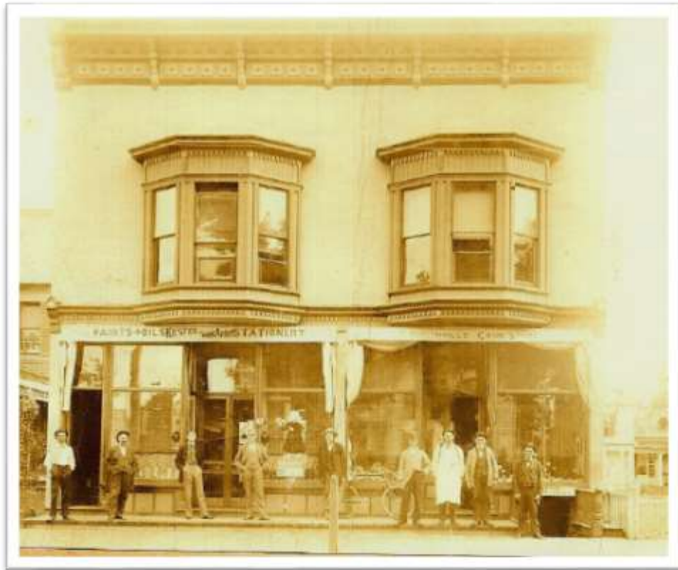
Kested and Cash Store date unknown (19 th c). Note entrance to the basement on right.
