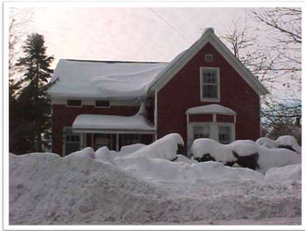
North Elevation (Façade)
