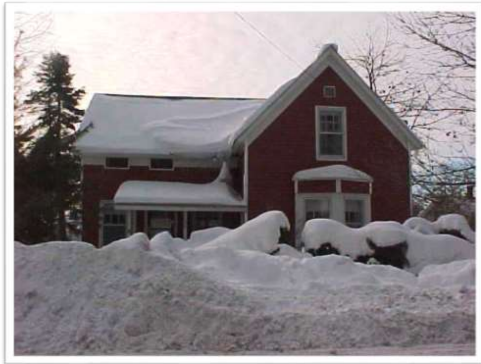
North Elevation (Façade)
