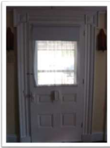
Interior door molding
