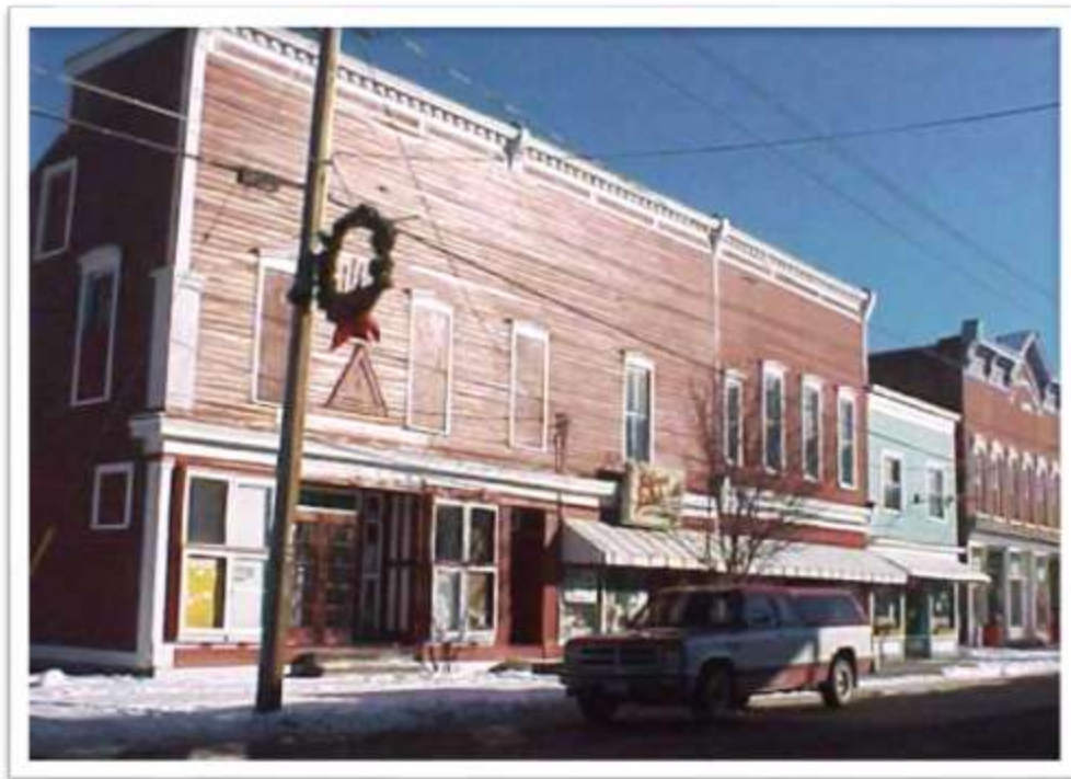
West Elevation (façade)
